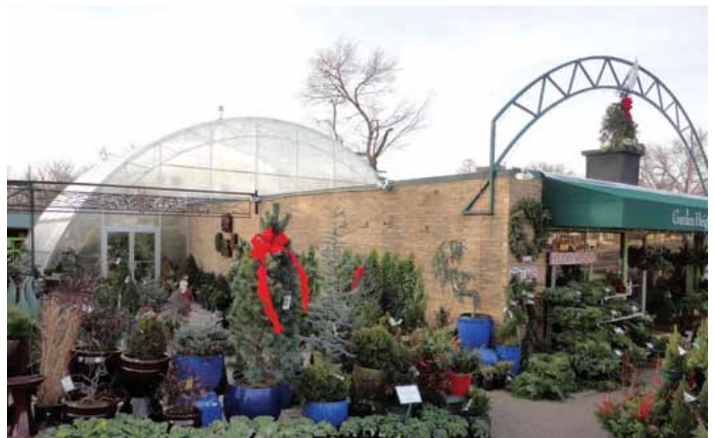
This new conservatory add-on to the back end of Garden Heights Nursery's original structure has given the retailer some much-needed interior space while creating unique and eye-catching look from the road.
