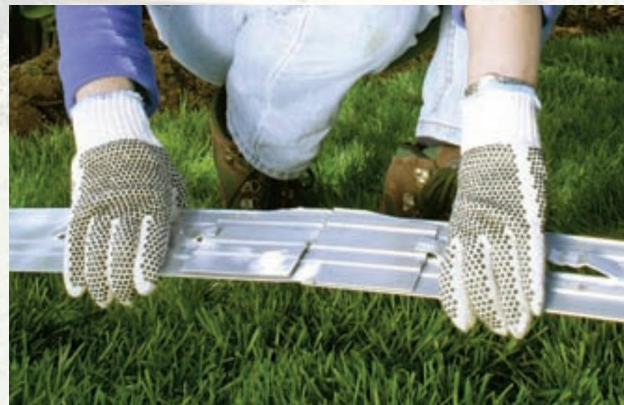
A permanent, stakeless connection system will provide the best performance, as well as speed up installation.
