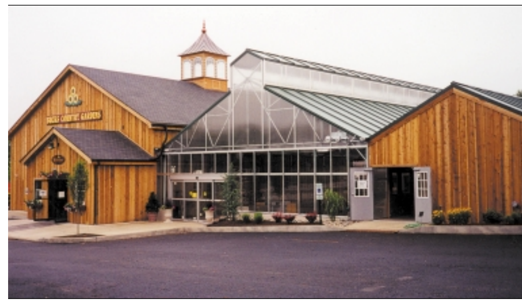
Bottom: Buck's Country Gardens, Doylestown, Pa., was built in 2000 by Nexus Greenhouse Systems. It is a Vail style with cupolas and vents, and there is a 2-inch metal span on the roof. Nexus Greenhouse Systems. (800) 228-9639. Write in 2021.
